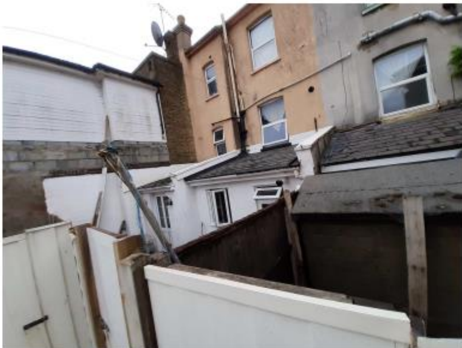
Neighbouring properties to the north-west
