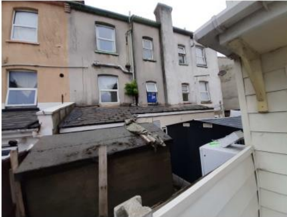
Neighbouring properties to the north-west
