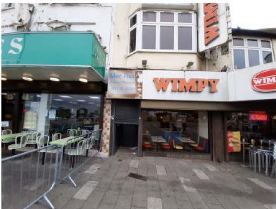
Entrance to the upper floors
